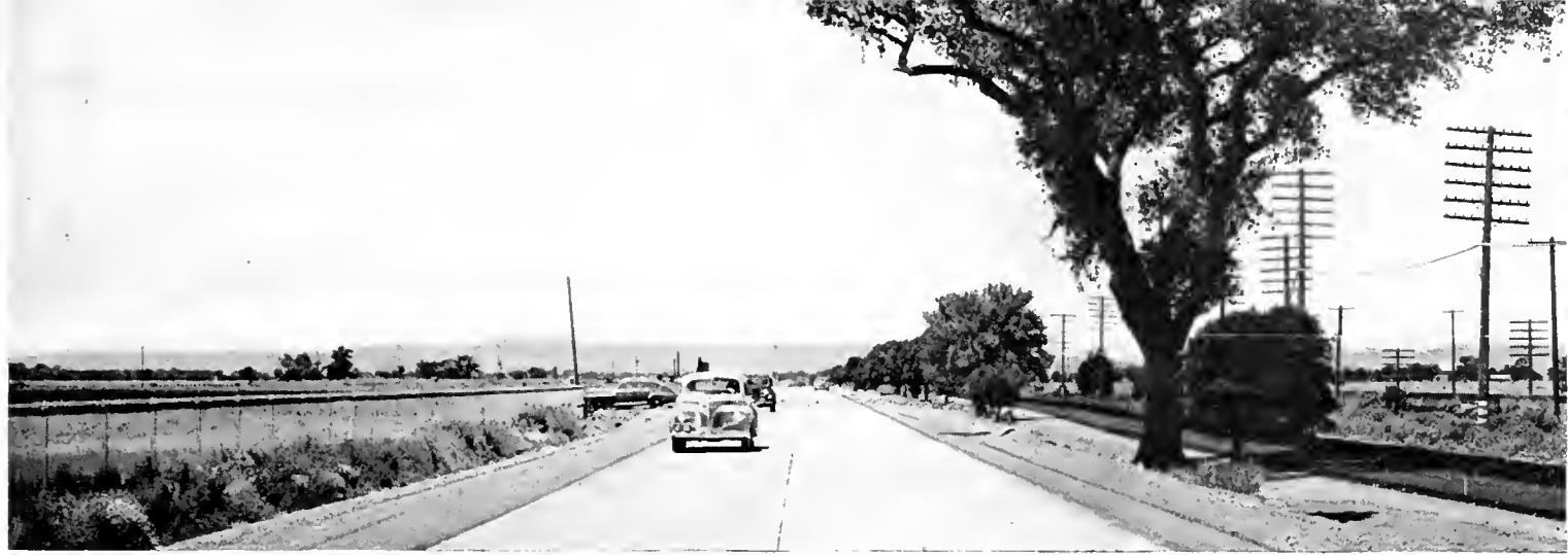
A 23-foot portland cement concrete pavement for one-way traffic on a recently completed divided highway section of U. S. 101
